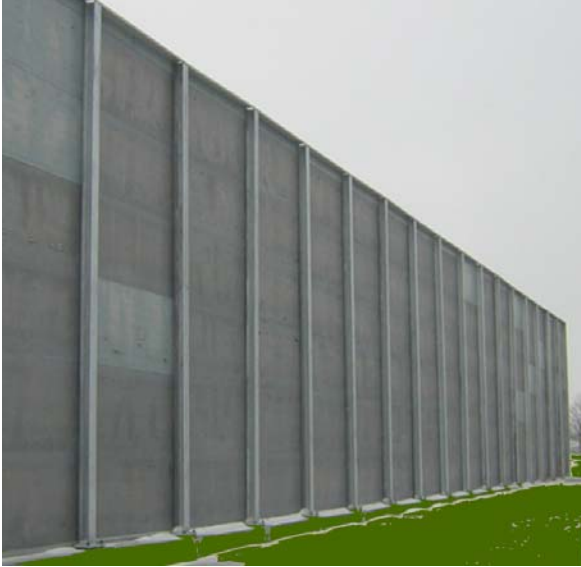
Airport Sound Barrier Wall
