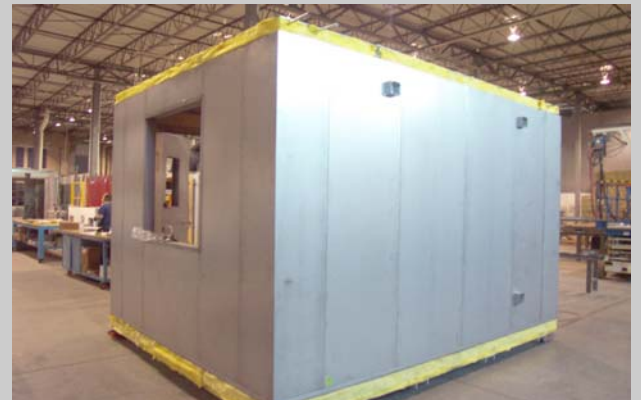
Assembled Structure Ready for Finishing Trim
