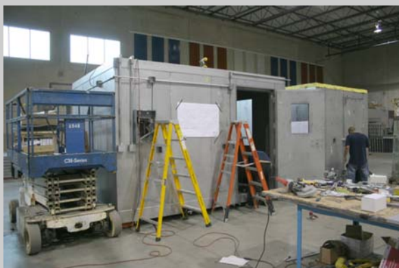
Electrical & Finish Work Being Completed
