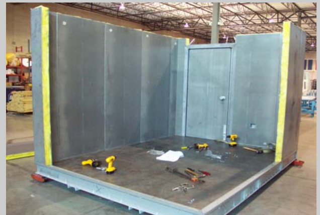
Modular Wall Panels Being Assembled Onto Base
