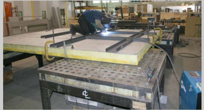
Custom Floor Section Being Fabricated
