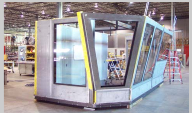
Custom Cantilevered Walls & Windows Being Assembled
