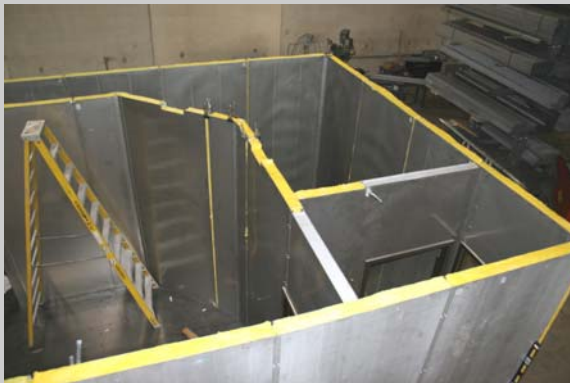
Custom Suite Being Assembled
