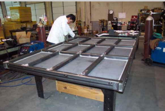
Custom Load Bearing Roof Section Being Fabricated
